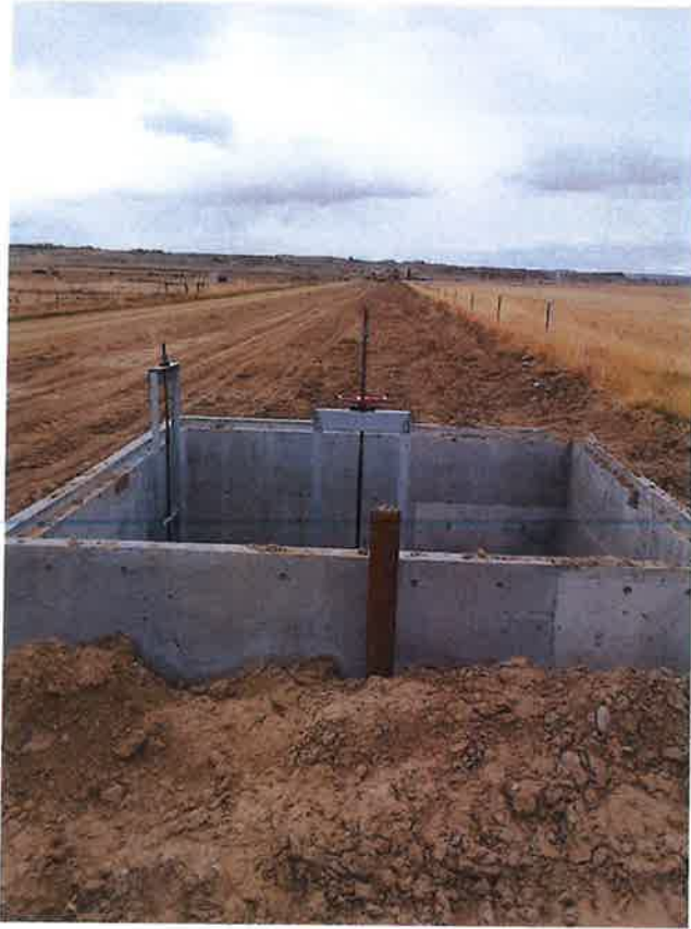
PM-5-Mile Pipeline & Structures
