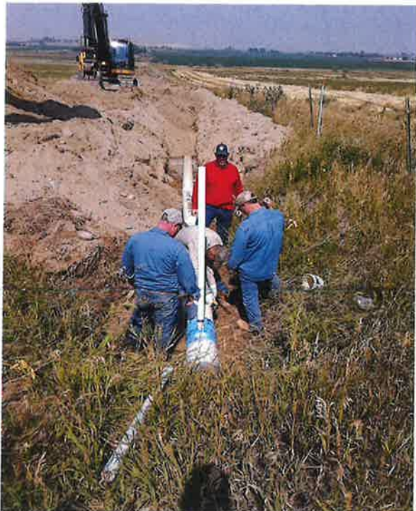
Devish Pipeline Project
