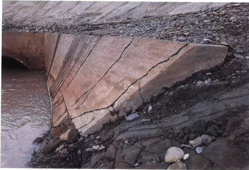
Pilot Butte Reservoir Inlet Wall Repairs
