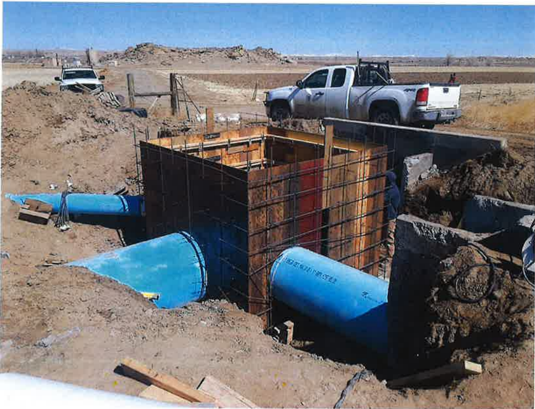
PM-5-Mile Pipeline & Structures
