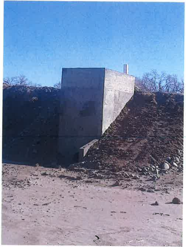
Whitlock Structure & Pipeline
