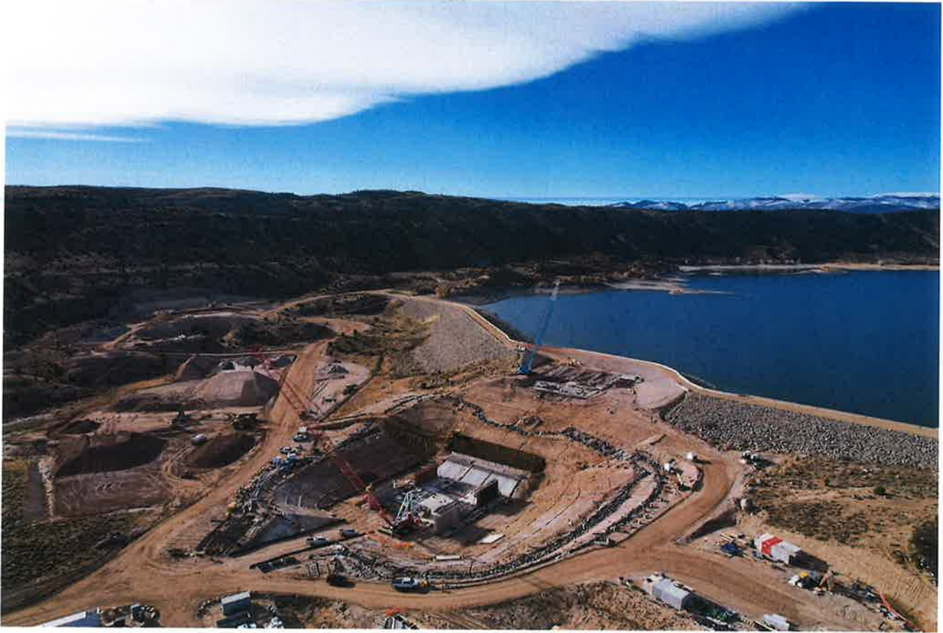
Bull Lake Emergency Spillway Project
