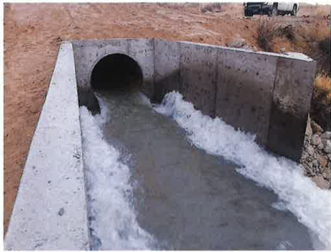
New Discharge Structure - Ocean Lake Drain at 5-Mile Creek
