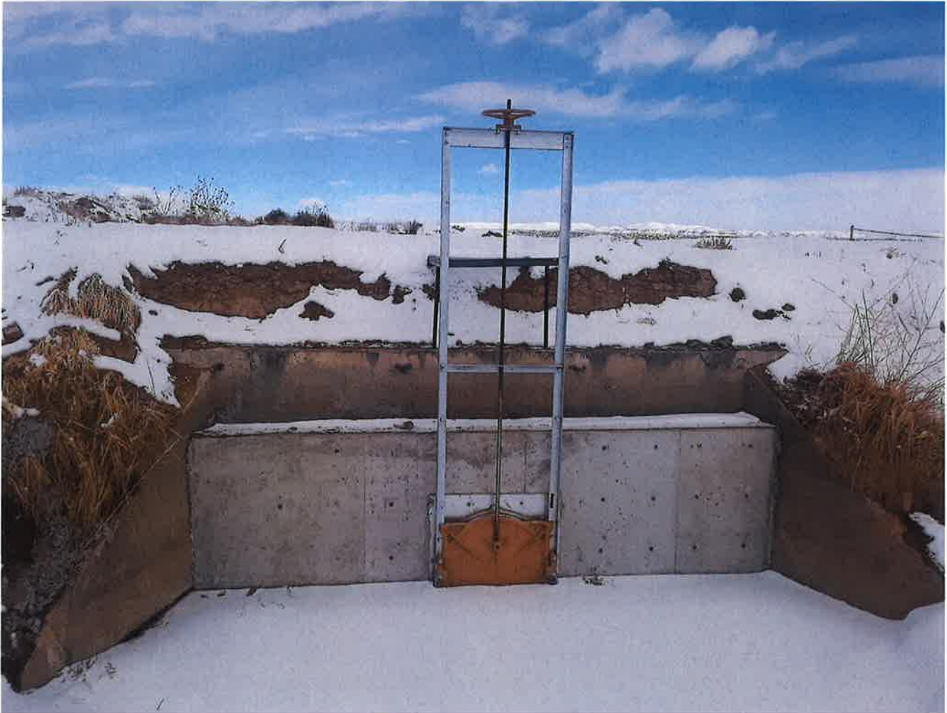
New 14.5' Headwall and 30" Headgate at Badger Wasteway
