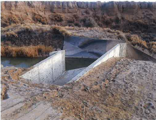
New Discharge Structure - Ocean Lake Drain at 5-Mile Creek
