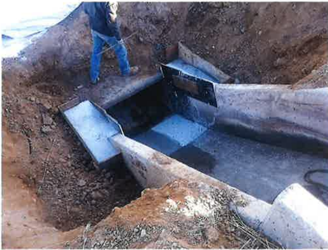
Existing Structure Repairs
