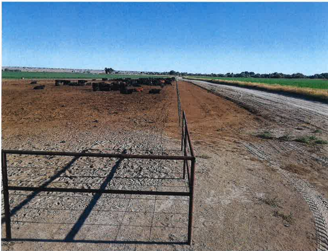
Midvale Encroachment Permits are critical to the protection of its facilities. (Above) Properly permitted fencing within PI-27.0 Piped Lateral easement.
