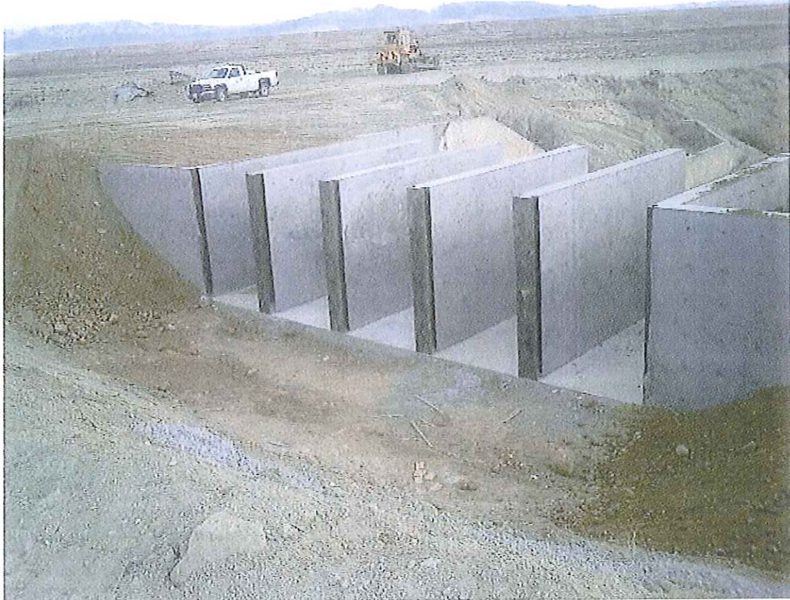
Wyoming Canal 37.2 Check Structure Replacement
