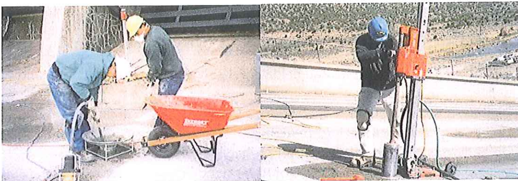
MIDVALE CREWS PERFORMING INTERIM REPAIRS AND CORING ON SPILLWAY SLAB
