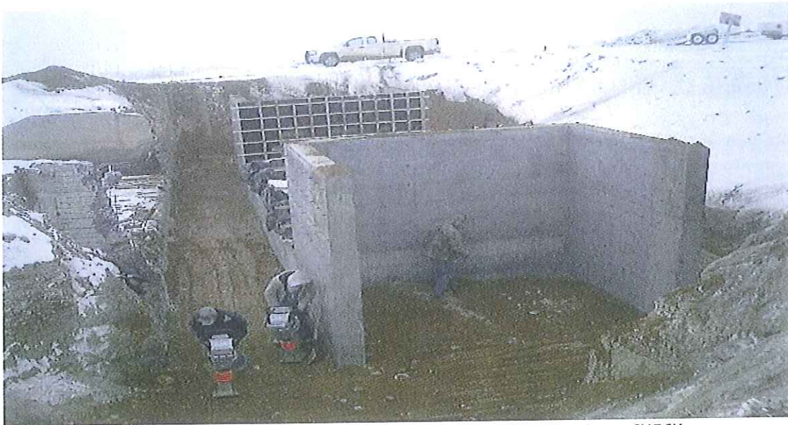
MIDVALE CREW COMPACTING BACKFILL AROUND NEW WC 37.2 CHECK
