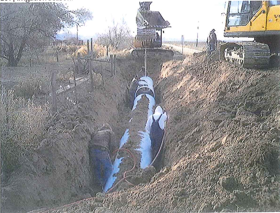
MIDVALE CREW INSTALLING 36" PVC PIPE on WC 15.1
