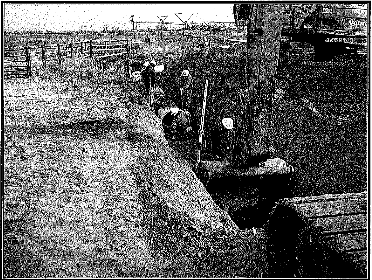
MIDVALE CREW INSTALLING 36" PVC PIPE
