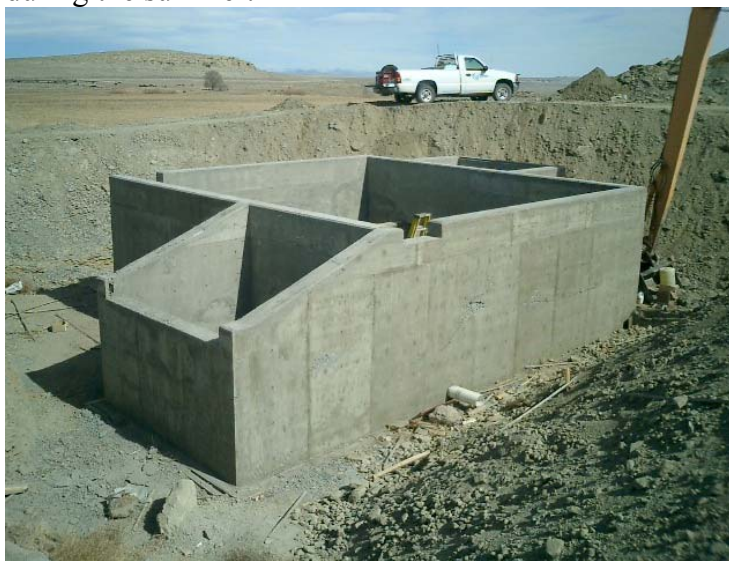
Hidden Valley Pipeline Inlet Structure
